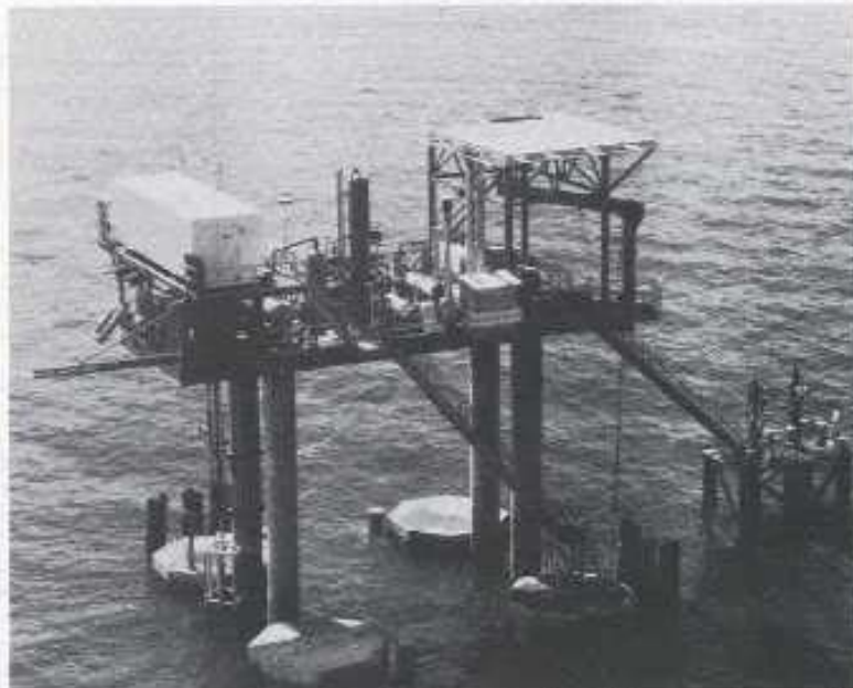
Seagull Energy E&P Inc.'s Eugene Island Block 45 production facilities are nominally rated for 20 MMscfd, but have handled up to 25 MMscfd and 60 bopd. Production equipment was installed on the steel deck at ground level and then lifted atop the barge.
